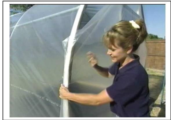
There are many different Poly Latching systems on the market from Wiggle Wire poly lock to Aluminum track lock. Most all of these must be installed over the top of wood frame for strength. Snap clamps are only recommended for smaller 10x10 or 12x12 portable garden units and are not recommended for larger in ground units. For use of our plastic snap clamps on small units please refer the specific unit you are building.
