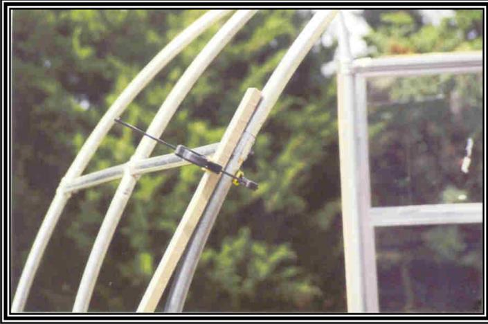
**Close up of bar clamp aiding installing strips. I soaked these strips in a nearby pond for several days before installing them so I did not need to kerf them.**
