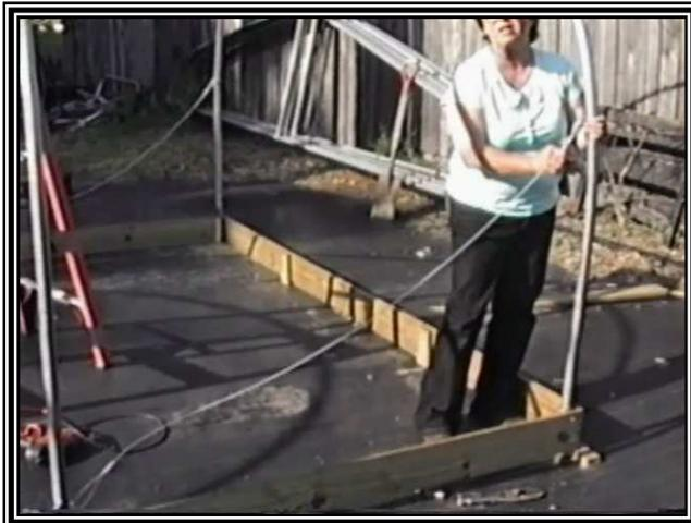
Here we are attaching cable to the end hoop at one end. Tighten the band clamp securely on the lower cable end at left and just snug up the band clamp at end hoop, leave some slack in cable for now. Install cables on opposite end same way
