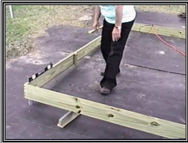
**Ground stakes are made of 1 5/8" fence post cut to 30 inch lengths. Loose soil may require longer stakes. As you can see we have already installed the ground cloth in a large area inside and out side of greenhouse. The ground is sloping towards this corner. After installing the 1 5/8 inch ground stakes I leveled the wood frame then blocked the frame up where needed to keep it level. Next step is to install the hoops.**
