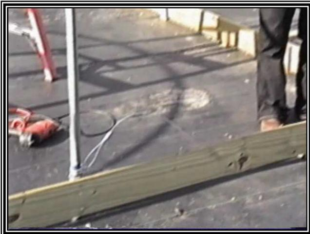
Here the cable brace has been clamped securely to the bottom of the first hoop back from each corner.
