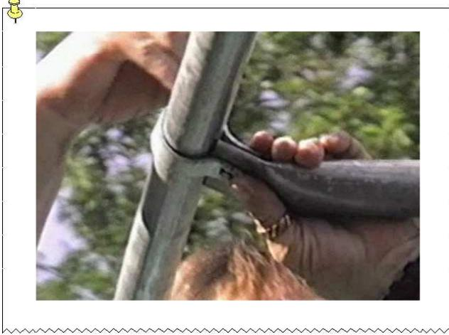
Attach the purlin at each end by flattening out the ends then bending the flat portion of tubing up about 30 degrees, drilling a 5/16 hole and using a band clamp made for 1 3/8" fence tubing. If you can not locate these fence clamps just make the purlin 1 3/8" longer on each end, flatten as shown, Holding the flat portion under the hoop and drill 5/16 hole thru the hoop and flatten end of purlin, then bolt with 2" X 5/16 bolt.
