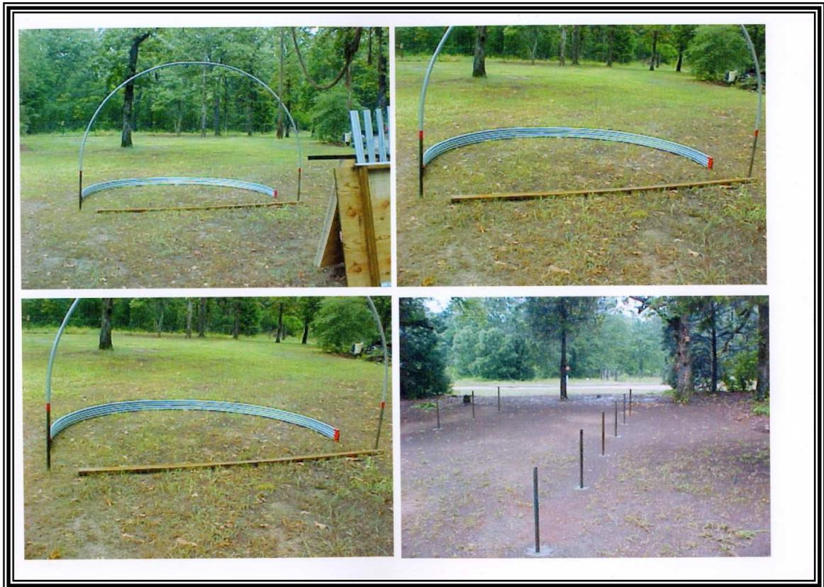
An alternate method for smaller in ground anchored greenhouses is simply build a sand box with 2x4s, level it, square it, then drive the stakes inside the sand box, using the box as a guide for stake spacing and alignment. Install hoops in stakes, fasten with tech screws from inside the greenhouse opposite the 2x4. After hoops are installed drill through the 2x4, stake & hoop and bolt them all together using 1/4"x4" carriage bolts or skip the drilling and use longer tech screws
