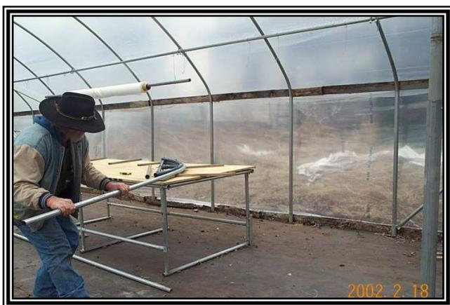
Here I'm completing the final bend on one section for a 12 foot hoop section. Note the already bent tubing being supported at the opposite end with the 1"x2" wood strips
