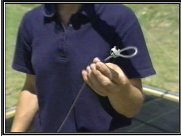
Here we have prepared the cable braces. Which are regular 1/8" steel cable from the lumberyard folded into a loop at each end and clamped with a 1/8" cable clamp also found at the lumberyard.
