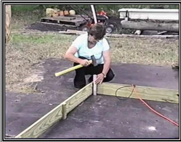
**Installing the last 1 5/8 " pipe stake corner stake.**
