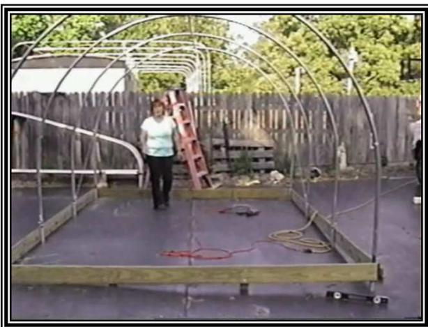
**The gap at front right corner will be filled in with treated wood later, leaving a screened outlet hole for water to escape the greenhouse. On longer house you may want to install stakes using a string line and level then hoops and add the wood band last.**
