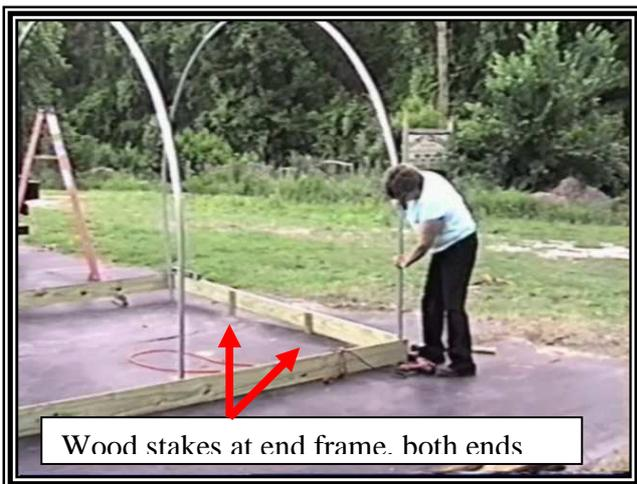
**Installing the last hoop. Hoops should be inserted into the 1 5/8" ground stakes 6 inches, then a #10 by 1 1/2" long self drilling screw is run through the wood into the 1 5/8" metal stake and hoop. This screw locks the frame in level position as well as connect the hoop to the stake. Two treated wood stakes at each end serve to stabilize the end frame boards. They are permanent so use treated wood.**
