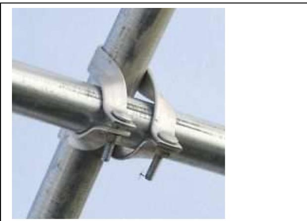
However we recommend using factory purlin clamps on greenhouse especially larger 16 ft or wider houses
