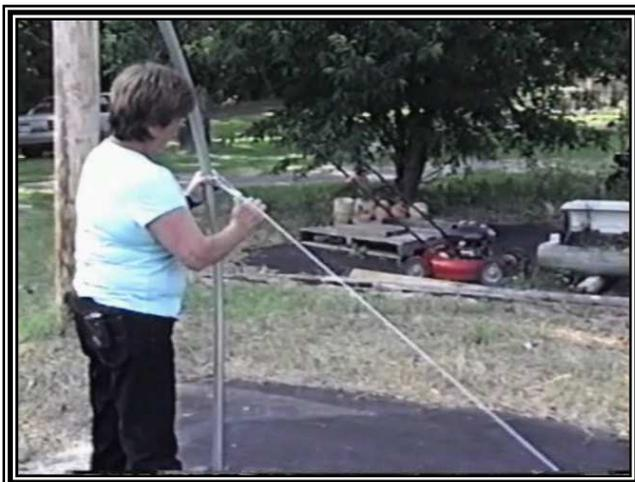
Sway braces can be made from the same tubing as used in the hoops, flatten the ends and bolt them in same locations as the cable braces, You will need to plumb up the ends first.
