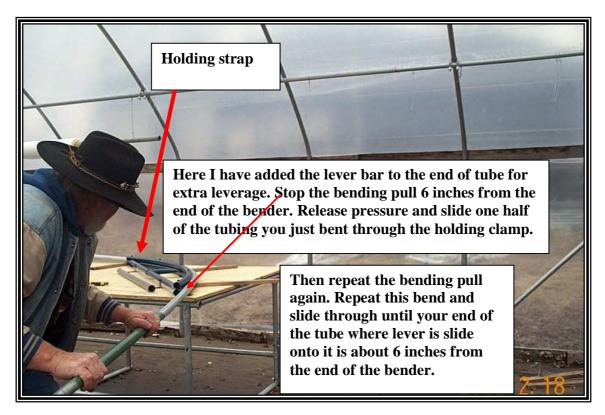
Always start the bending with the painted ends inserted through the holding strap. In the case of bending the 12 ft. wide hoops you will push the painted ends of all tubes 4 inches past the holding strap. Never place the un-pained ends into holding strap.
