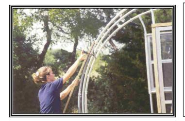
Clamps can be used to hold 1x2 wood strips as the are bent around the end hoops. Remember only the end hoops get the 1x2 strips. If wood is hard to bend, you can kerf the strip. This is simply cutting across the strip about 1/3 through every 1 to 2 inches.
