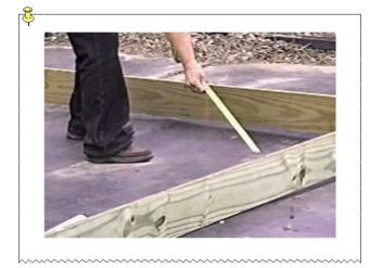
Shift side "B" left or right until you get five feet between the two marks on the diagonal measurement. It's then square, Provided that you have cut all four of the side boards to their required length, if one board is wrong then the frame will not square up...
