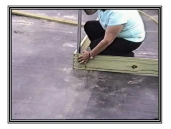
Install the self drilling (Tech) screws from outside wood into the 1 5/8" stake and hoop
