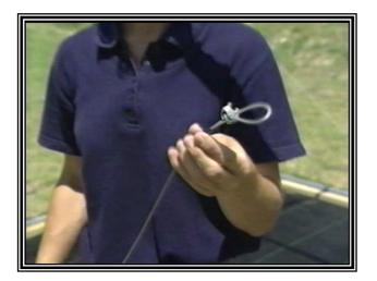
Here we have prepared the cable braces. Which are regular 1/8" steel cable from the lumberyard folded into a loop at each end and clamped wit a 1/8" cable clamp also found at the lumberyard.
