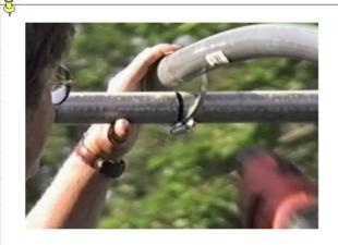
Attach the perlin at each end by flattening out the ends then bending the flat portion of tubing up about 30 degrees, drilling a 5/16 hole and using a band clamp made for 1 3/8" fence tubing. If you can not locate these fence clamps just make the perlin 1 3/8" longer on each end, flatten as shown, Holding the flat portion under the hoop and drill 5/16 hole thru the hoop and flatten end of perlin, then bolt with 2" X 5/16 bolt.
