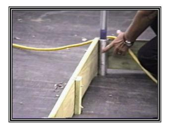
Pushing the hoop down into the 1 5/8" O.D ground stake. Here you can see the top of painted end. Top of paint is 6"
