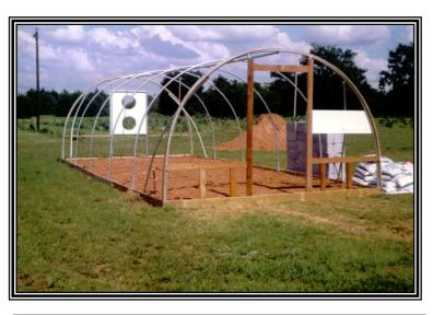
Another customer supplied photo. A great example of a very clean professional job preformed by the homeowner. Note the holes for twin exhaust fans in rear. He used tubing framing for end walls but bolted wood to front end wall for easier door installing.
