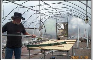
Here I'm completing the final bend on one section for a 12 foot hoop. Note the already bent tubing being supported at the opposite end with the 1"x2" wood strips
