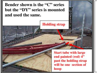
Remember the 12 wide frame is a two piece (section) hoop. The photo at left shows placing one of these 10'6" tubes with large end painted red into bender, When you bend the other half section tube you will push the small end painted (red) through the holding strap 4". And bend as instructed. When both sections are completed they will join together at the top of the hoop,described later.
