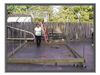
The gap at front right corner will be filled in with treated wood later, leaving a screened outlet hole for water to escape the greenhouse. On longer house you may want to install stakes using a string line and level then hoops and add the wood band last.
