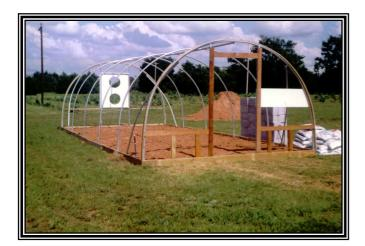
This is such a good example of GH construction I had to add it again. Note also the earth grade work inside the frame work. Slightly raised above outside grade.
