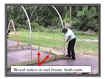
Ground stakes are made of 1 5/8" fence post cut to 30 inch lengths. Loose soil may require longer stakes. As you can see we have already installed the ground cloth in a large area inside and out side of greenhouse. The ground is sloping towards this corner. After installing the 1 5/8 inch ground stakes I leveled the wood frame then blocked the frame up where needed to keep it level. Next step is to install the hoops.
