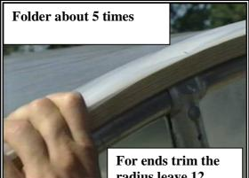
For ends trim the radius leave 12 inches extra to fold and staple onto the 1x2 strip right over the top plastic staples
