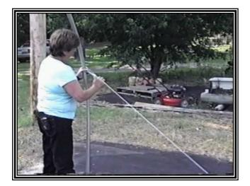
Here we are attaching cable to the end hoop at one corner. Tighten the band clamp securely on the lower cable end at left and just sung up the band clamp at end hoop, leave some slack it cable for now.
