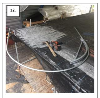
The completed hoop is still in the bender. This one was bent on our LT-4 bender. However the bending steps are always the same except the distance from the end you start bending.
