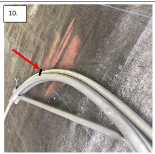
After pushing the bent tubing through the clamp another 8" or 10" and bending that short third stroke, you can see how much closer the 5' mark is to the clamp than in photo #9. Now remove the entire tube from the bender.
