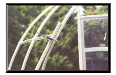
Close up of bar clamp aiding installing strips. I soaked these strips in a nearby pond for several days before installing them so I did not need to kerf them.
