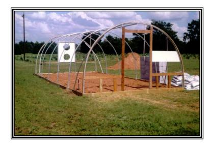
Another customer supplied photo. A great example of a very clean professional job preformed by the homeowner. Note the holes for twin exhaust fans in rear. He used tubing framing for end walls but bolted wood to front end wall for easier door installing.
