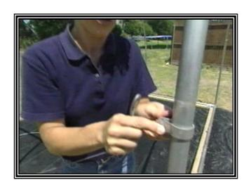
Here we are using those handy 1 3/8" fence band clamps. Any chainlink fence supply can order these clamps if you can't find them. Also some success has been noted using heavy metal plumbers tape with holes punches in it. Or solid tubing braces can be used, cut the tubing to desire length flatten the ends and tec screw it to the inside of hoops at the four corners. In place of the cables
