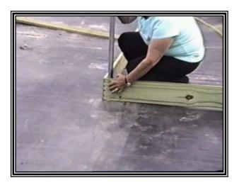
Install the self drilling (Tec) screws from outside wood into stake and hoop
