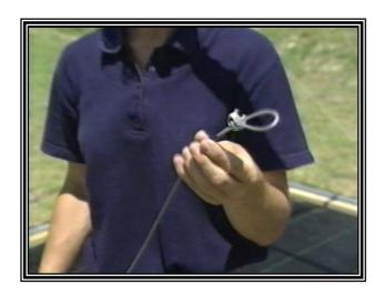
Here we have prepared the cable braces. Which are regular 1/8" steel cable from the lumberyard folded into a loop at each end and clamped wit a 1/8" cable clamp also found at the lumberyard.
